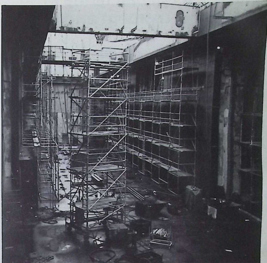
Mounting longitudinal bulkheads
