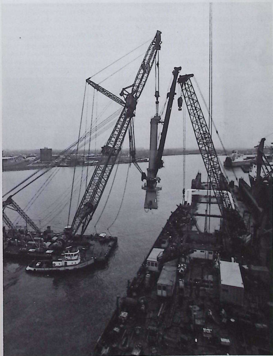
Heavy Lift Mast Crane installation
