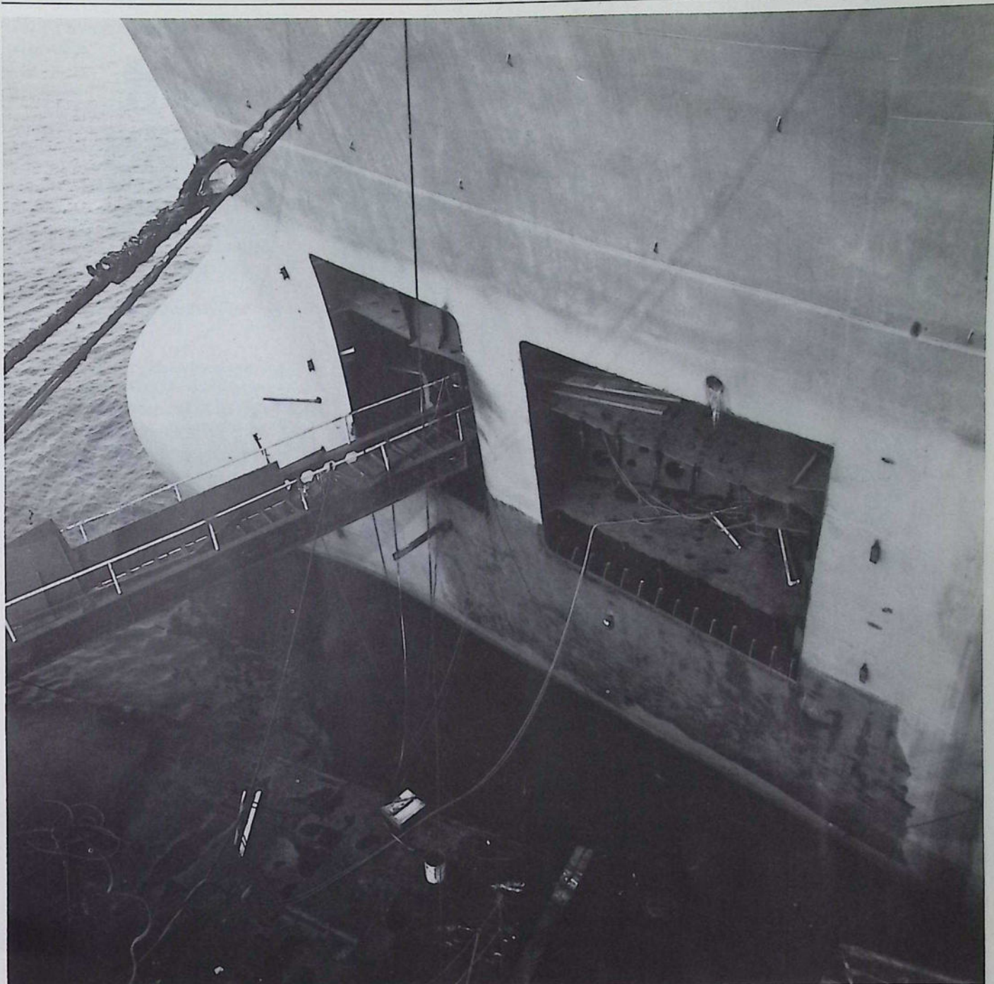
Temporary front entrance
