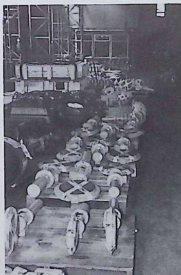
(Duvalco Butterfly-valves complete with Cupedo hydraulic actuators ready for shipment to Boele Bolnes)
