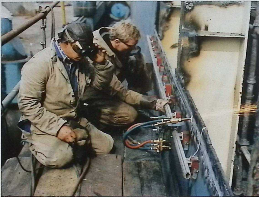
▲ Modern bevelling of hull plate during extensive repairs on ro-ro vessel „Matina”, owned by UBEM S.A., Antwerp.
