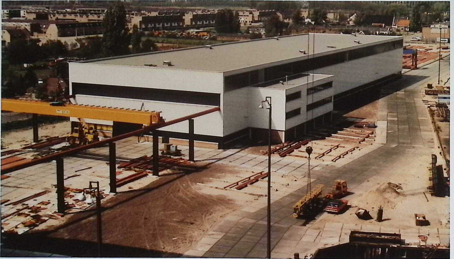
▲ A new plate shop of 117 × 30 metres.
